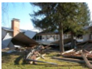
Slika 7. Razkrito ostrešje osnovne šole v Ribnici (foto: Simona Fajfar/Delo) Figure 7. Uncovered roofing of Primary school in Ribnica (Photo: Simona Fajfar/Delo)
